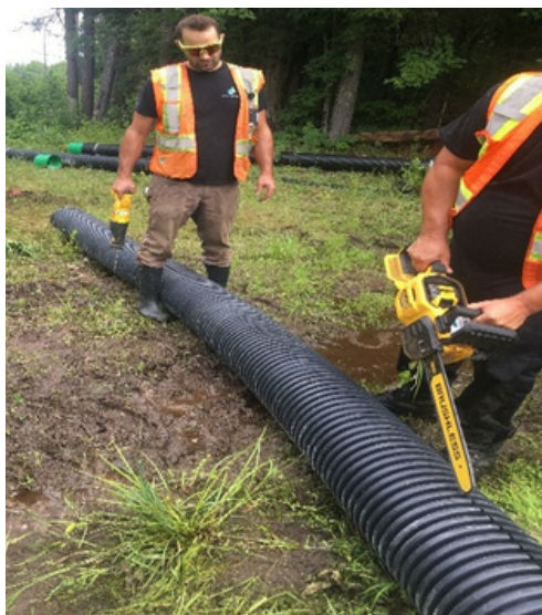
FIGURE 1.5: Perforation des anneaux du drain flexible perforé
